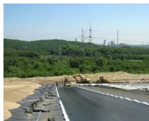
Picture 4: Geomembrane Panel Deployment
