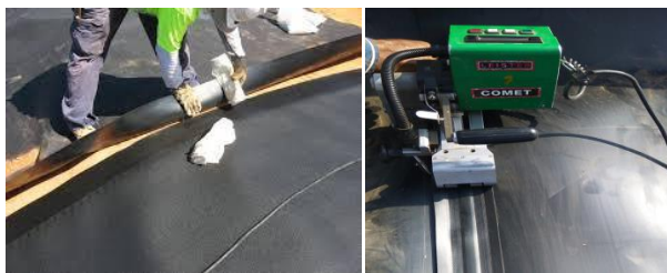
Picture 7: welding of geomembrane
