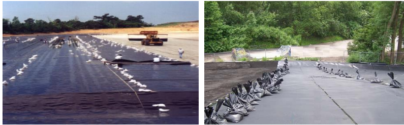
Picture5: hold the geomembrane with sand bag in position
